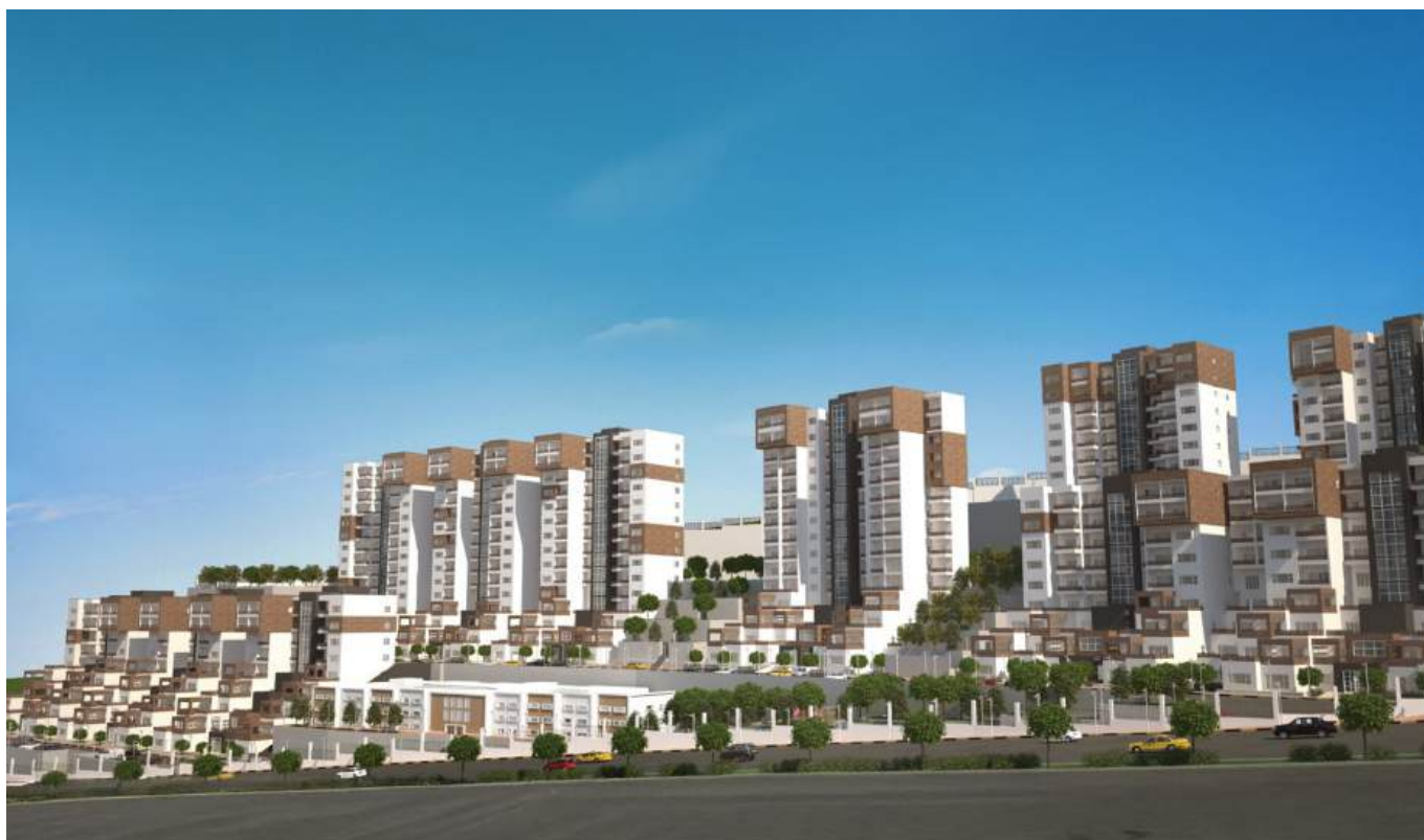
Project Name : Daik City City : Suleymaniyah / Iraq Date : 2023
