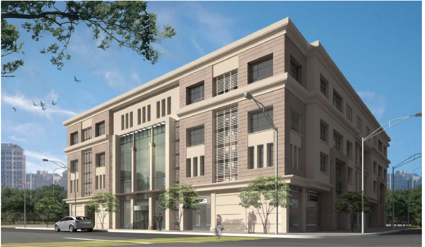
Project Name : Applied Syndicate Building City : Tanta / Egypt Date : 2021
